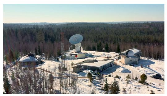
Metsähovi Geodetic Research Station. The gravimetric laboratory is at the left, the new VGOS radio telescope in the centre and the SLR observatory at the right. Behind it is the new main building.
