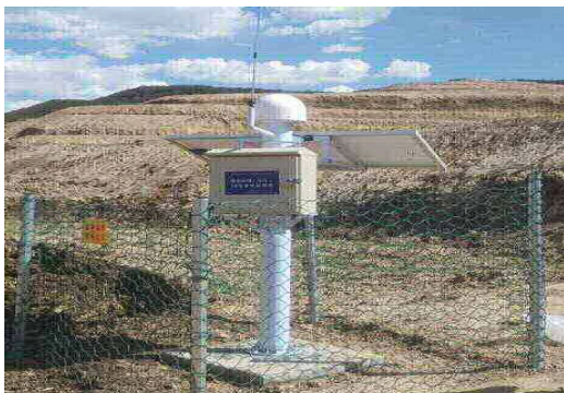
Sensor installation for Cloud Platform for SHM and Warning at engineering sites in China
